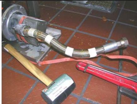
Fig 4: Pump after discharge piping converted. Reapply heat tape to flex hose when finished re-piping pump outlet.
