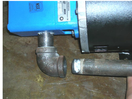
Step 22. Apply thread sealant with fluoropolymer (kit item 4) to both ends of 3/4" space nipple and to end of pump inlet nipple with pump inlet coupling. Attach 90 degree 3/4" npt elbow and 3/4" npt space nipple (kit item 2) to pump inlet port as shown using an adjustable pipe wrench. Assemble nipple with pump inlet coupling to 3/4" 90 degree elbow using adjustable pipe wrench.
